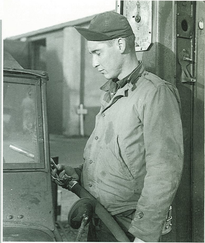
Above: This driver will "fill 'er up" from a gas pump outside the Motor Pool Office which was located on the Tech Site. The pump, minus many components, and quite dilapidated still stands today. (96th Archives)
