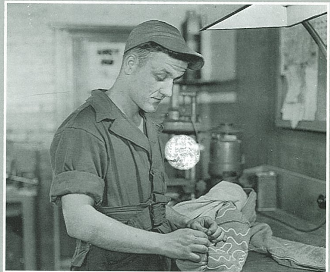
Sgt. Musser carries out inspection and repair on an electrically heated flying suit. In early days these suits proved unreliable, as the heating elements were wired in series and failure of one section of element would result in total failure of the whole suit. The heating element is clearly shown here in white on the blue woolen suit. (Daniels & Kueppers)
